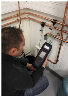
DHW network temperature
