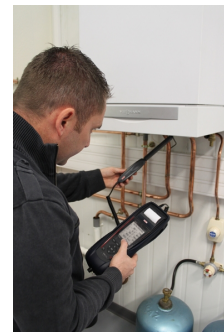
Ambient CO checking
